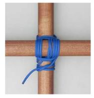
Tighten the lashing by surrounding it with three or four frapping turns. Finish with two or three tight half hitches.
